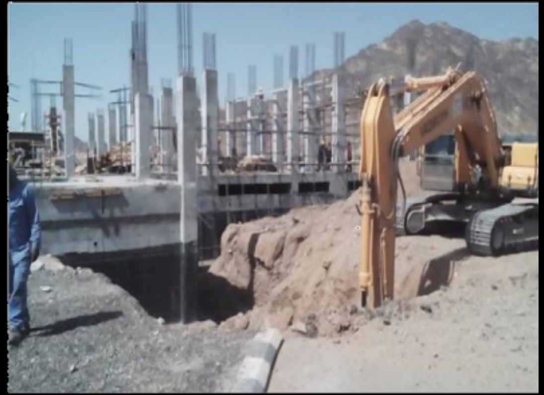
Progress works at Al Khatam 110 KV
