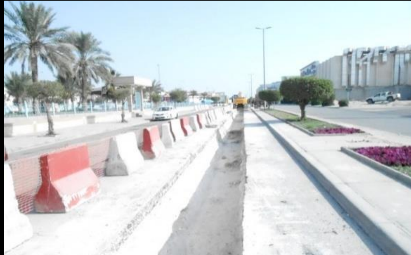
Installation of cable works for KAPP 115 K
