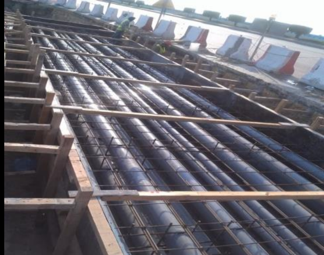
Steel Fixing For CBD at Section 20 on KAAP
